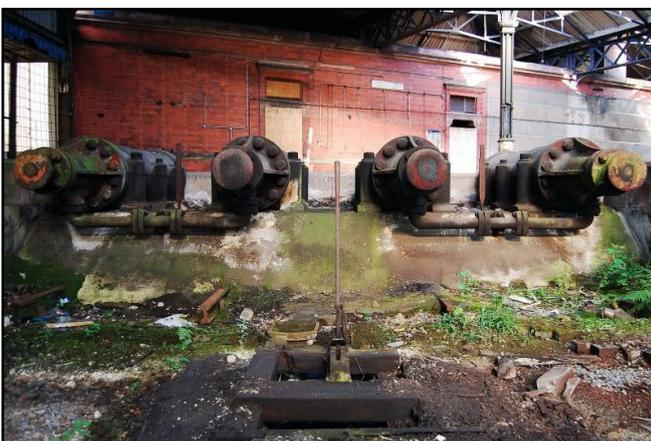
End of platform buffer stops. The lever in the middle was to release "trapped" engines after uncoupling. It's a wonder the scrap metal boys haven't got this lot.
